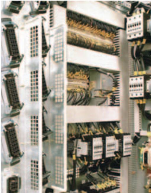
All the train's control signals come together in one control cabinet. This is connected externally by means of heavy-duty plug-in connections. Our space-saving Z series terminals, MCZR TRAK-type relay couplers and diode holders maintain an electric connection and ensure that the signals in the control cabinet are analysed reliably.
